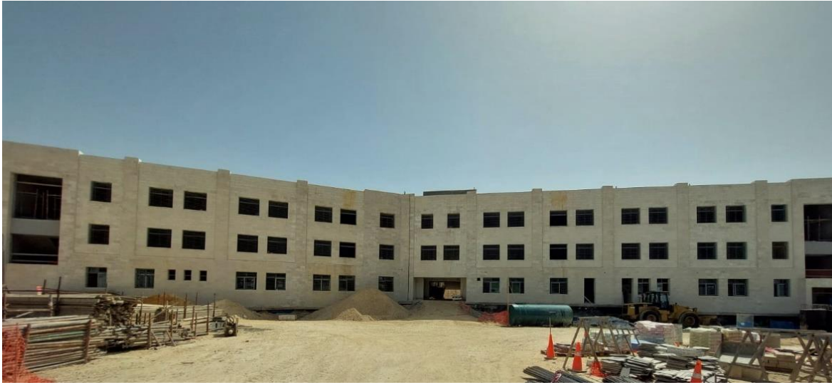
General view of the project site
