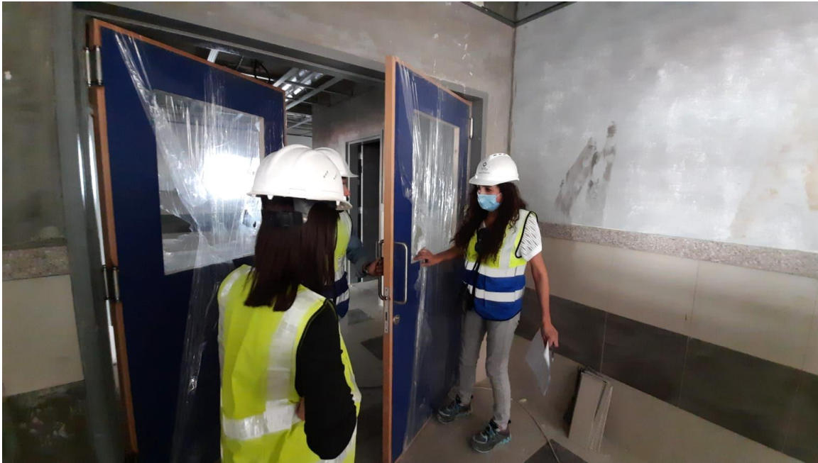
The team inspected the installed swing doors in the corridors
