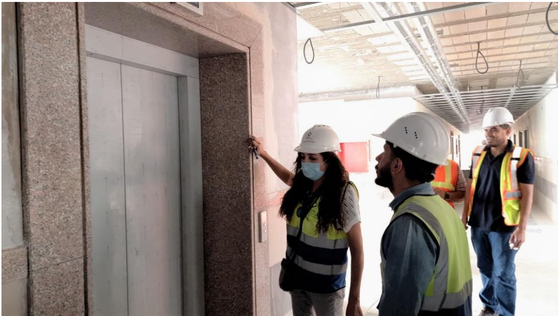
The team inspected the installed accessories for the elevator
