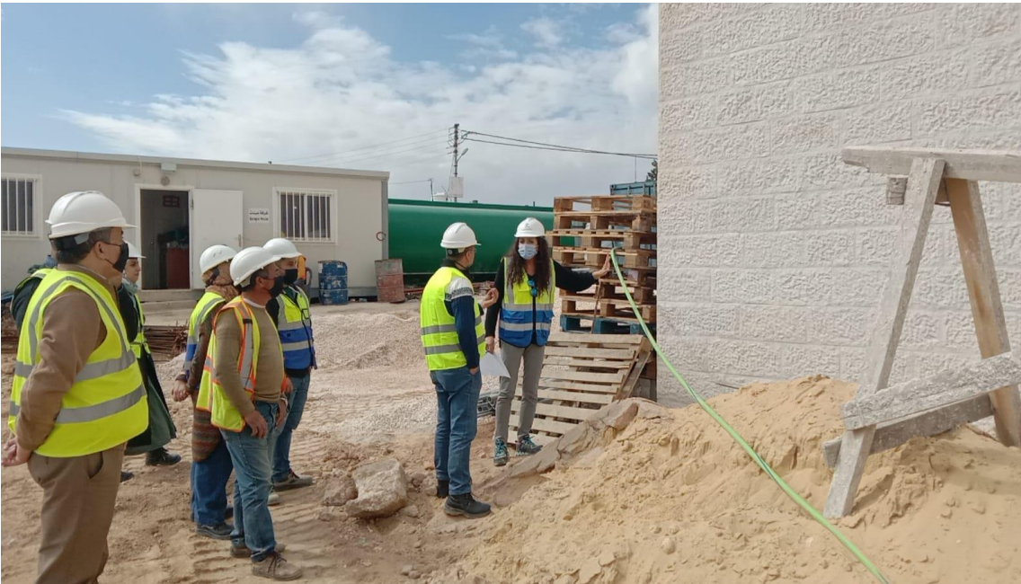
The team inspected the stone facades of the building
