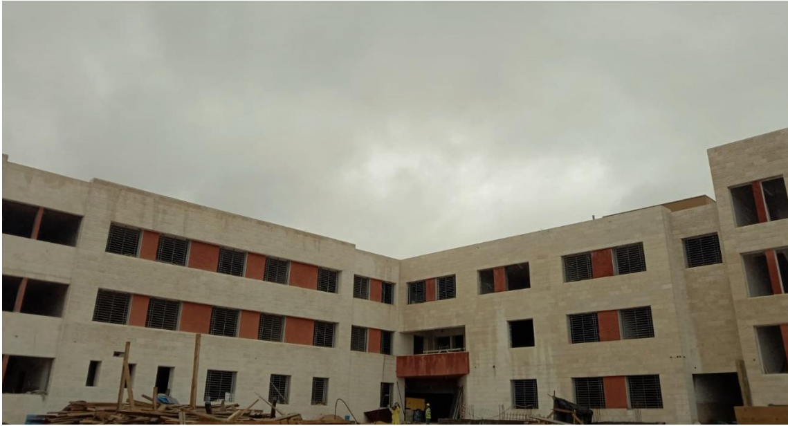
General view of the project site (Figure: 01, 02 & 03)
