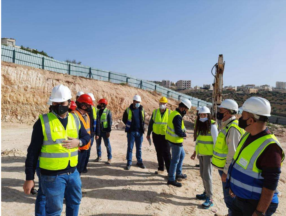
All parties discussing the preparation stage of the shoring system
