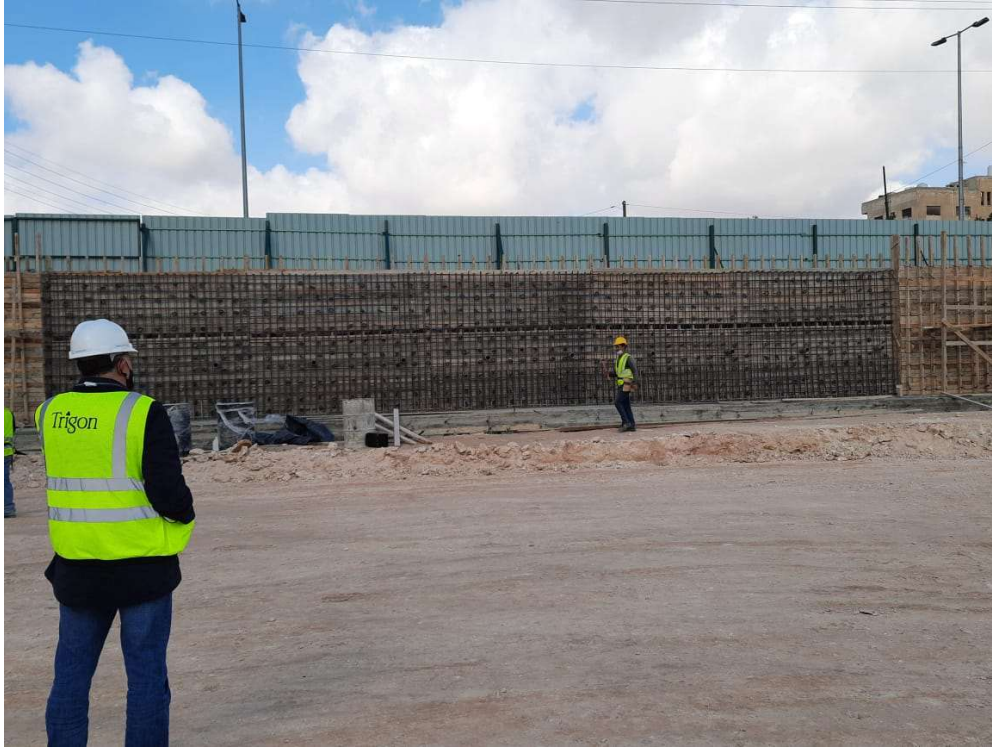
Eng. Osama Watching Boundary Wall Works
