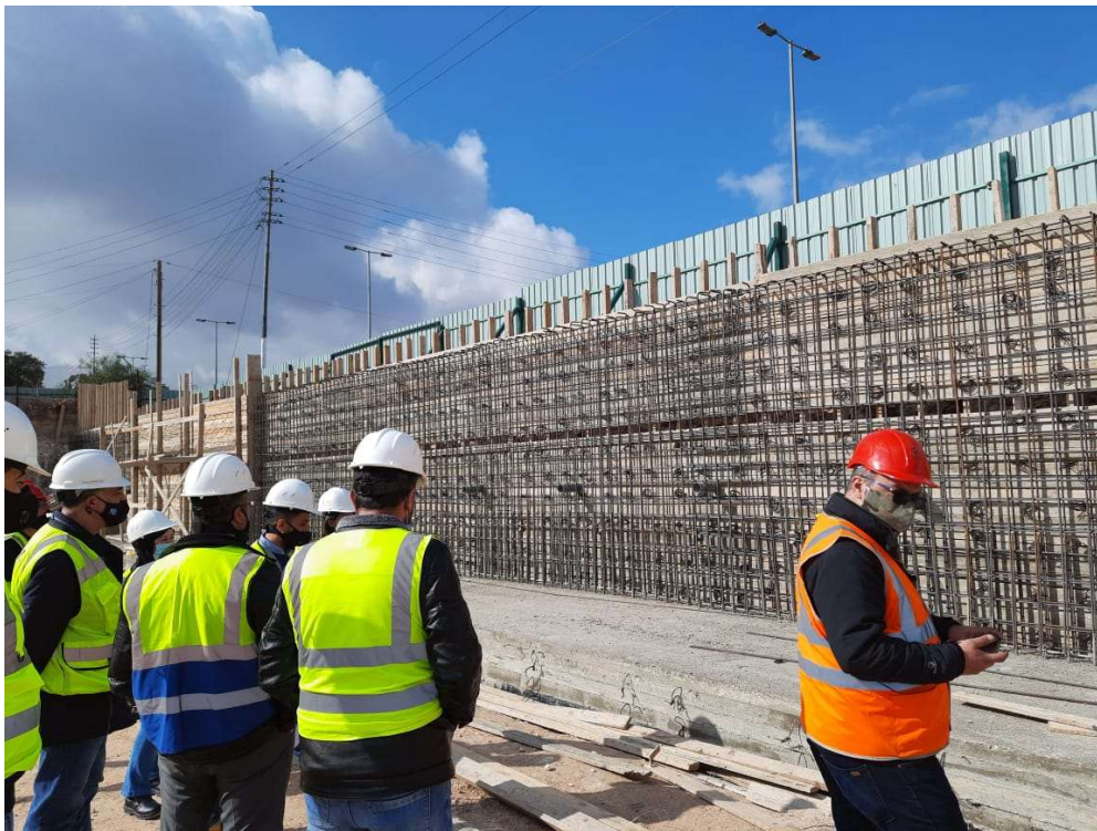
Work in boundary walls
