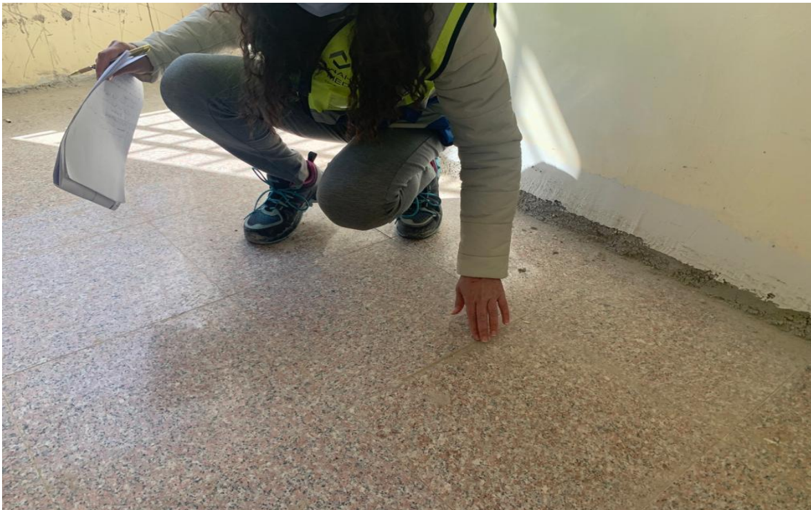
Teething in the granite tiles for landing
