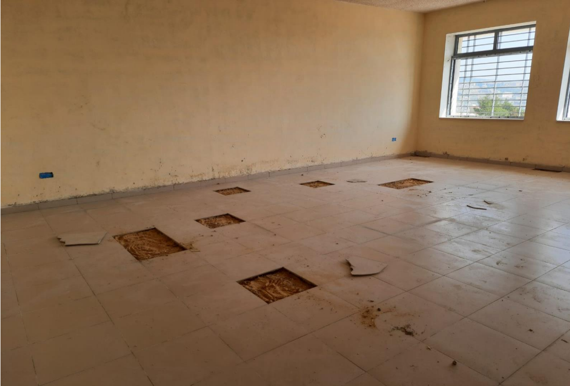
Removing of defected porcelain tiles
