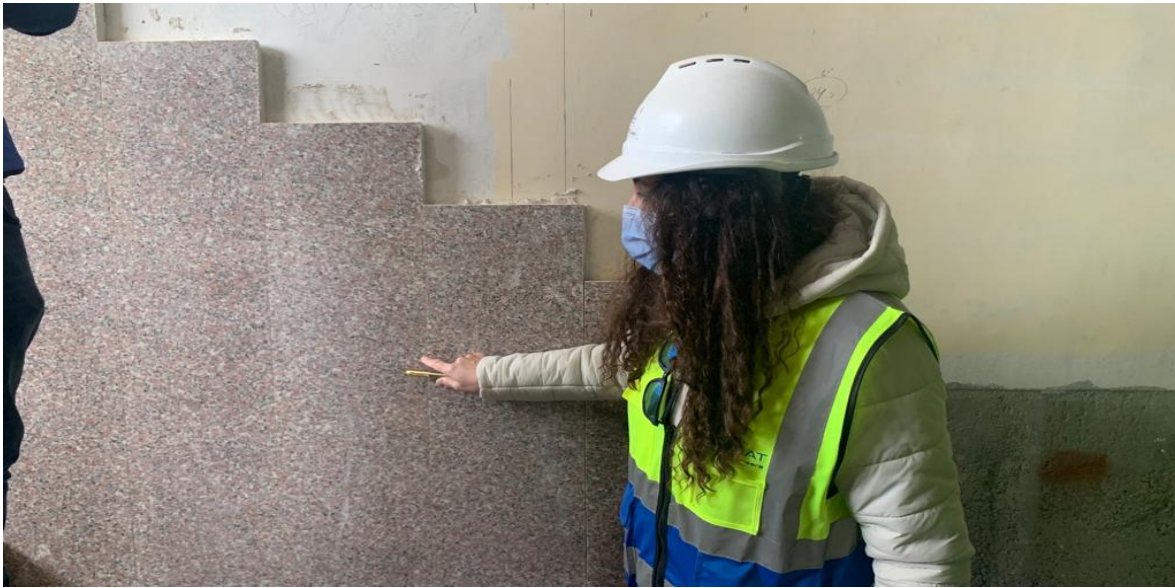
Teething in the granite cladding for staircases
