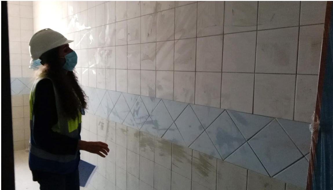
Inspecting wall tiles at the wet areas
