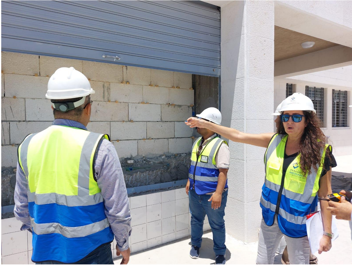
The team observed defects in the executed stone for the water fountain
