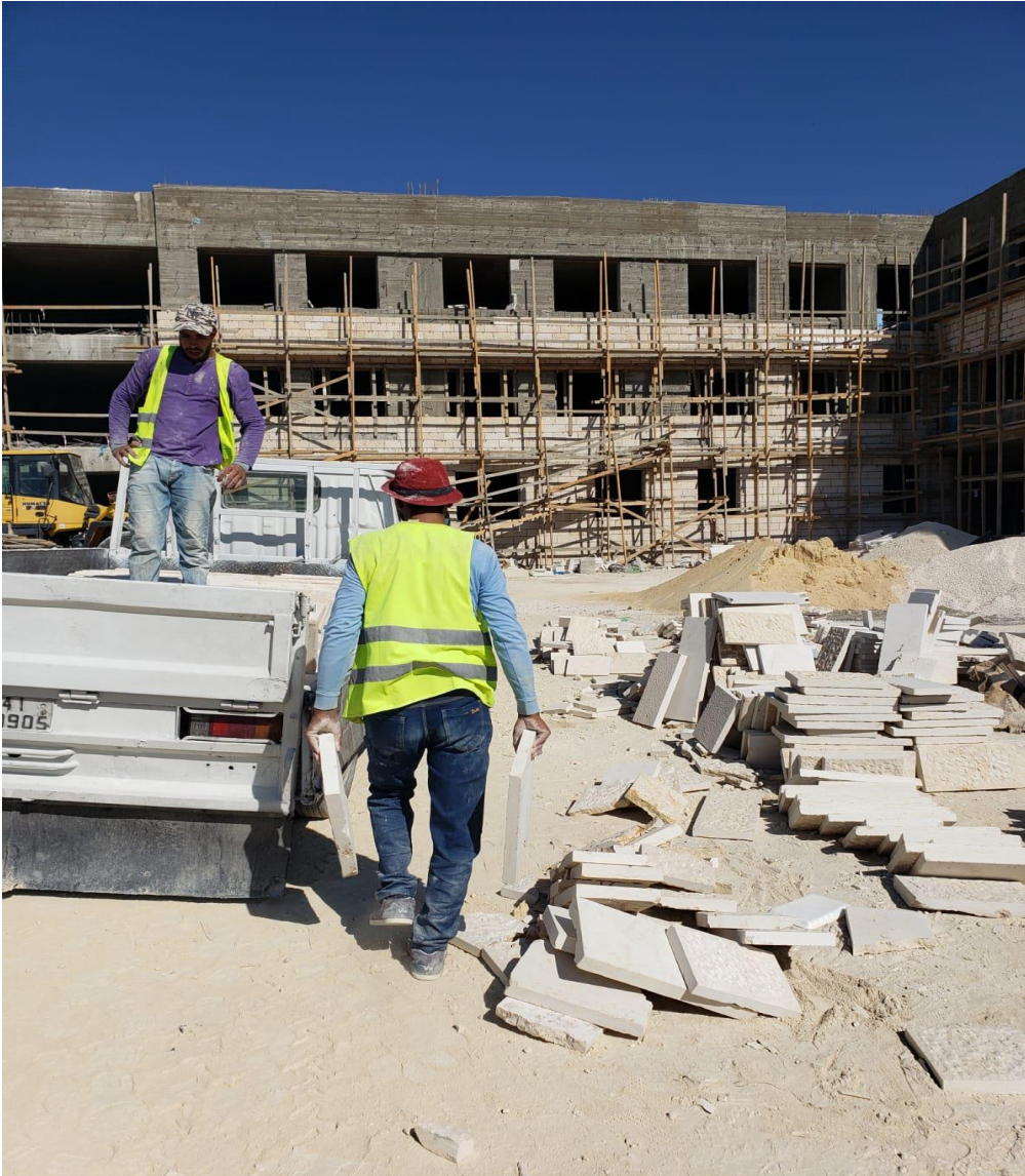
Removing Un- Complied Stones Outside the Site
