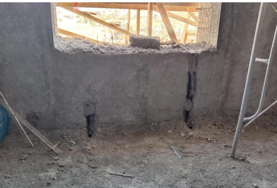
Radiators: Execution of first fix (Bottom-Top) without approval
