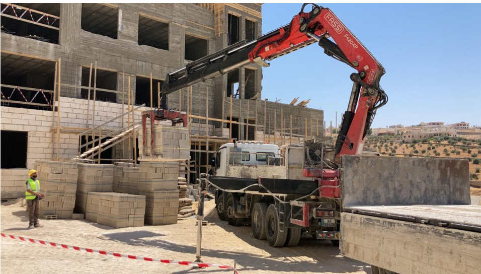
Delivering hollow block to the site
