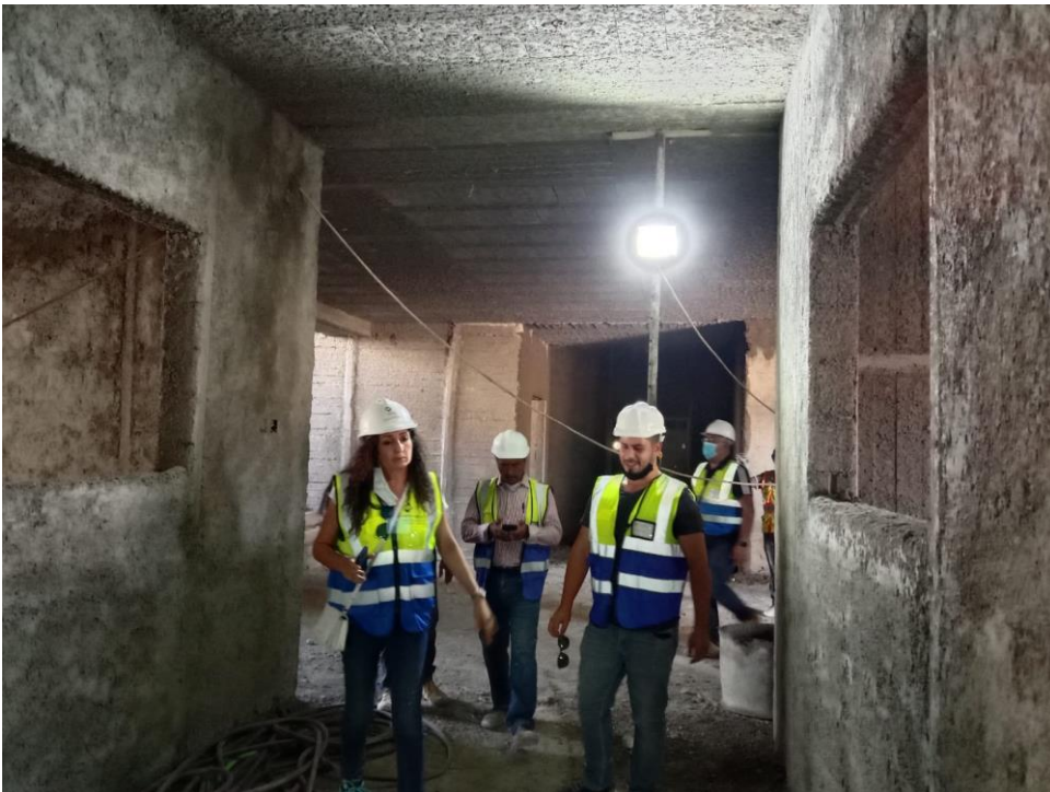
Acceptable process and quality for plastering work
