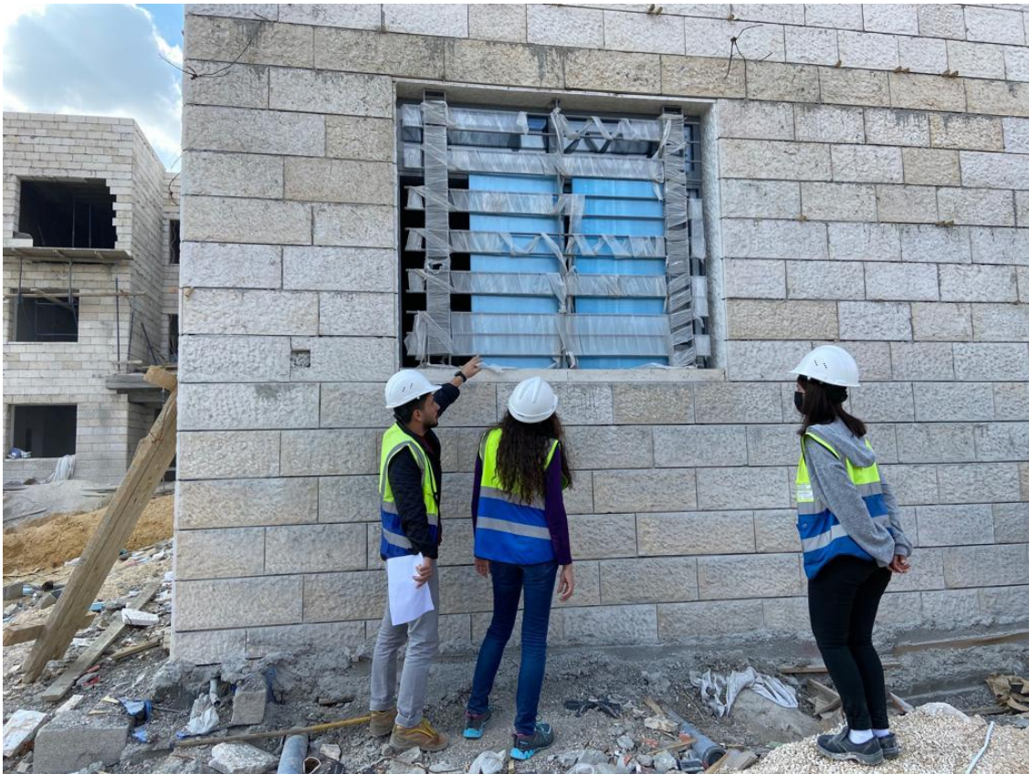
The sample of window protection grill was inspected and approved
