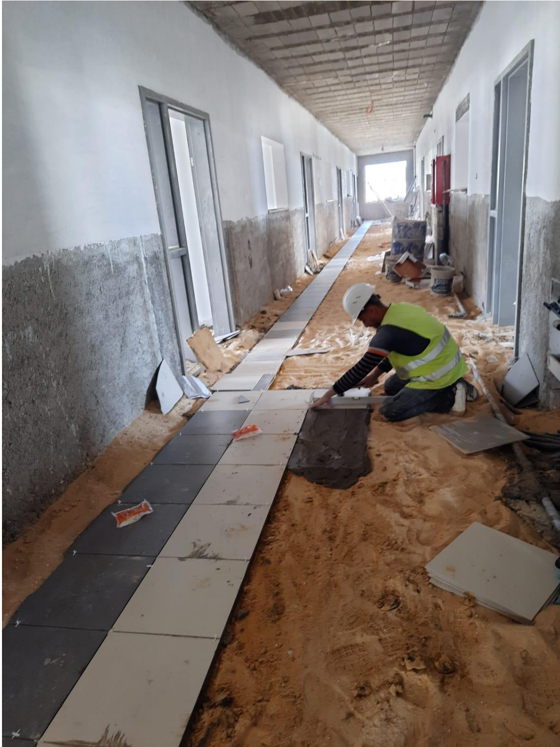
Tiling work at the corridors
