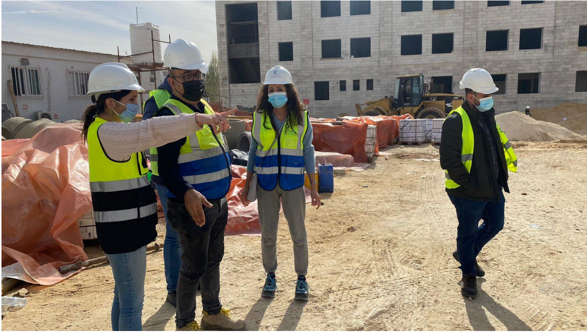
Medanat site engineer/Eng. Saba gave a brief about the ongoing activities
