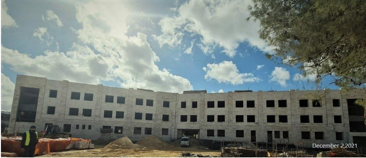
General view of the project site
