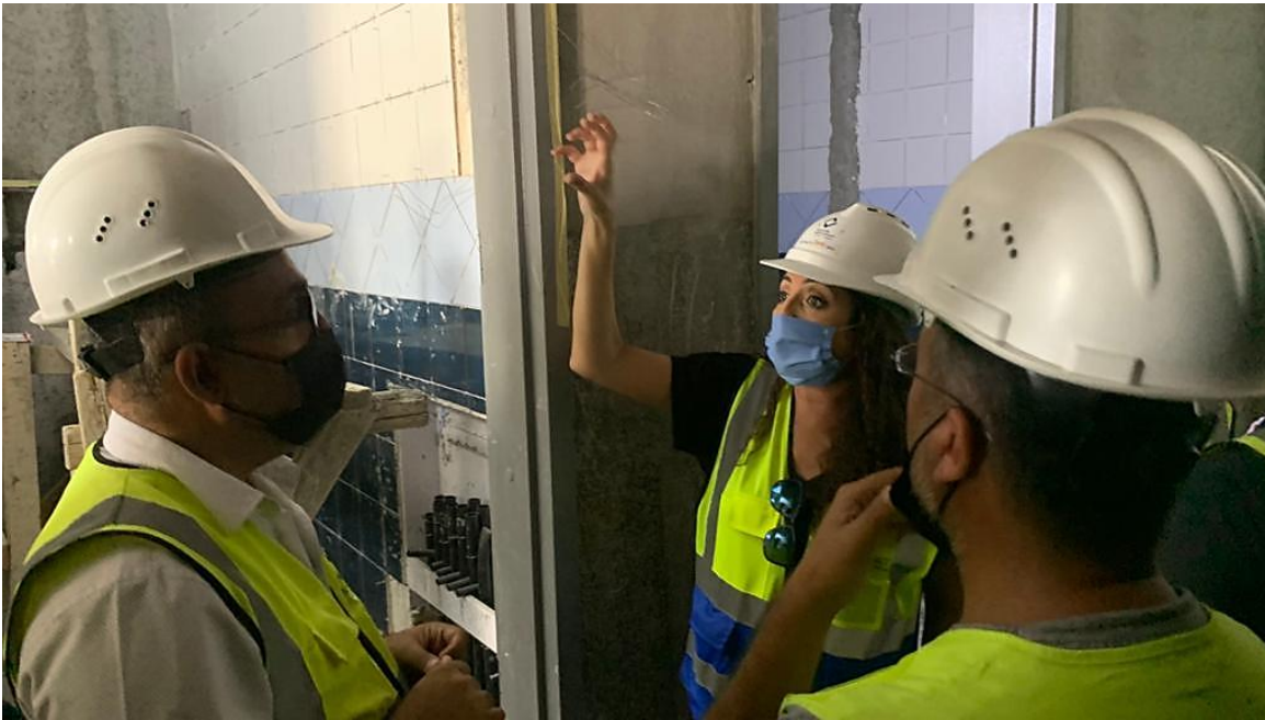
The relationship between the door frames and the wall tiles of the sanitary units was discussed
