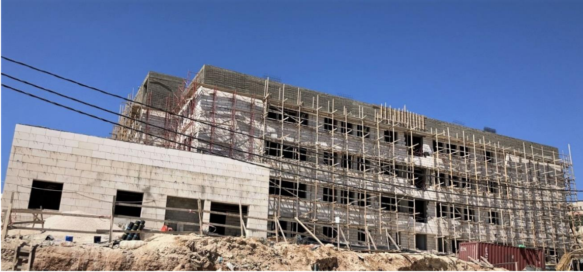
General view of the completed third floor casting (the last slab)
