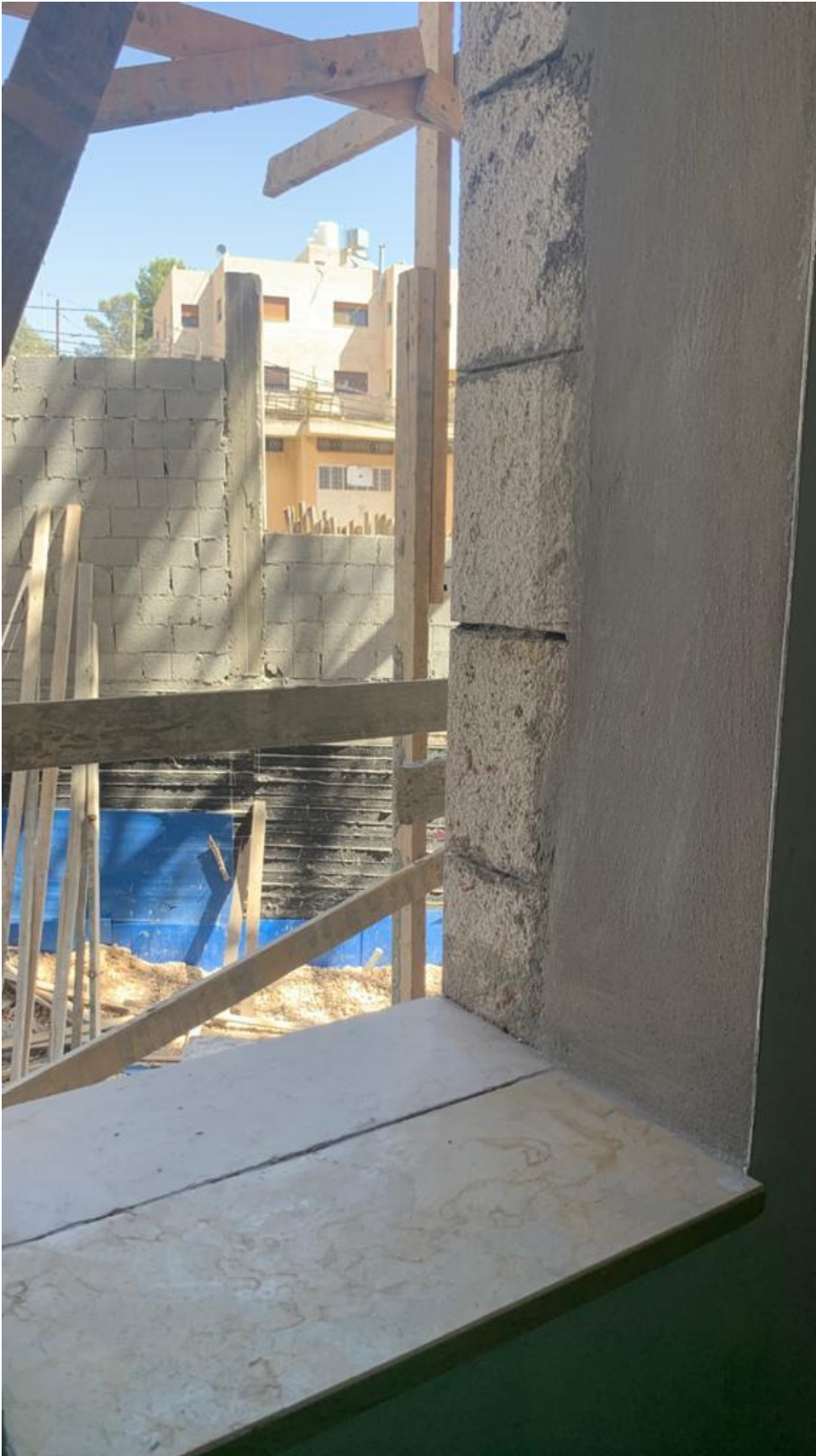
Installing window sills and jambs finish as per requirement
