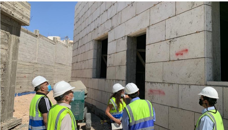
Checking quality of stonework
