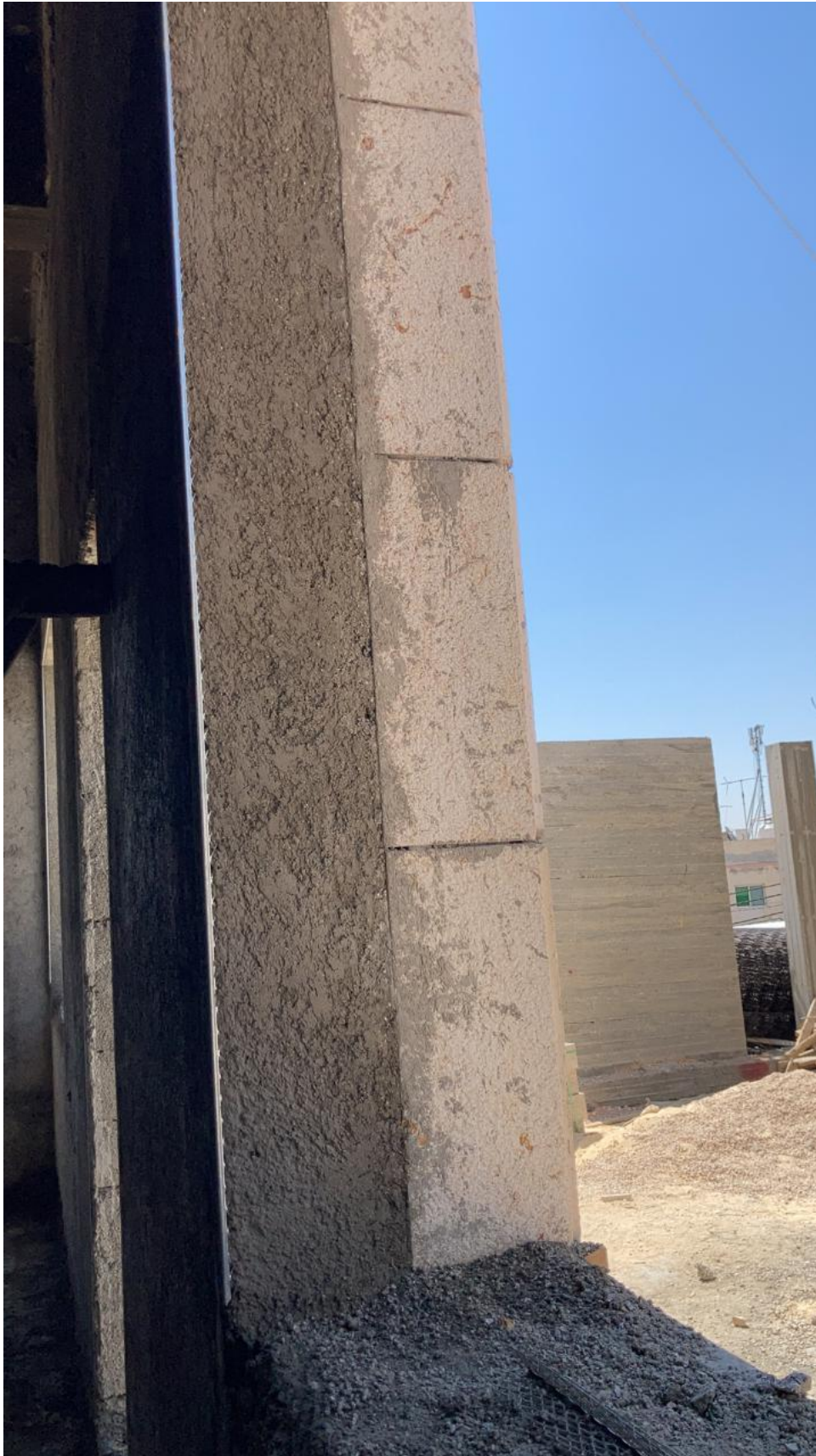
An example of the concrete jamb for windows as required
