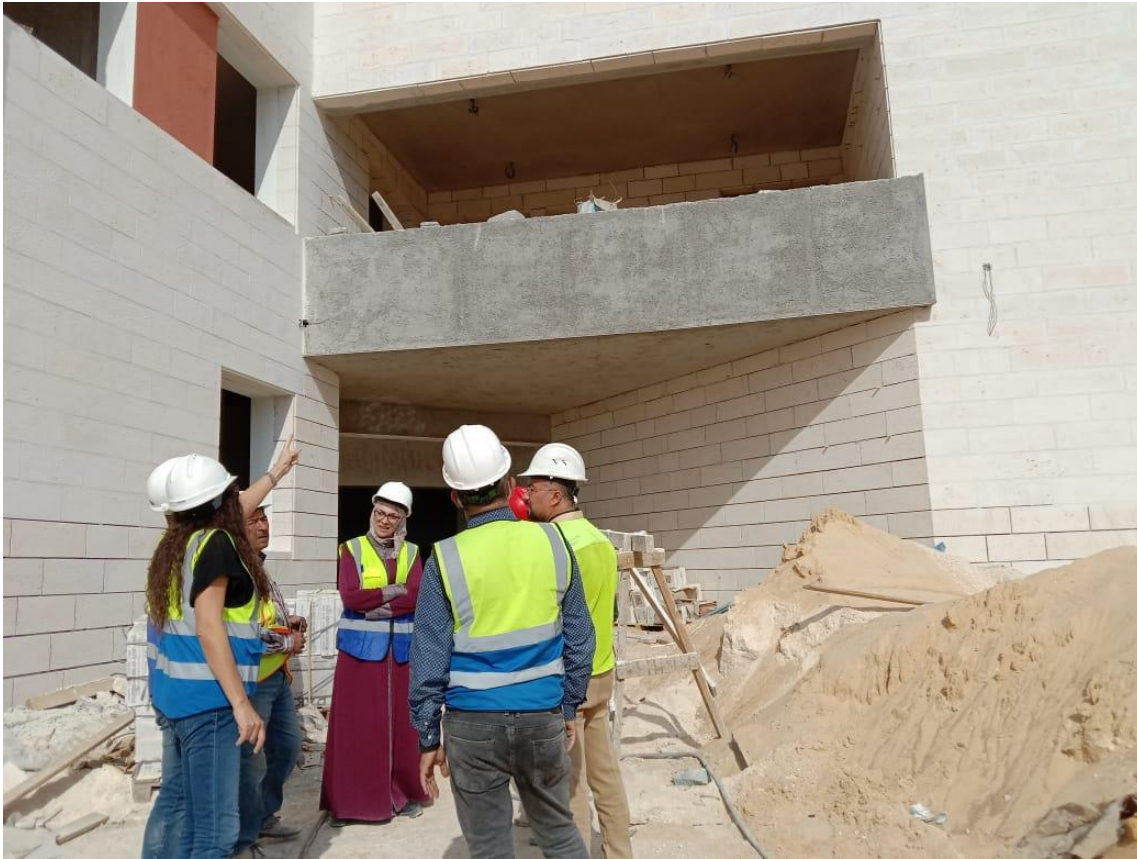
Discussing the entrance canopy final finish
