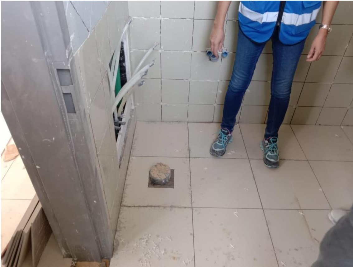
Installing floor drain according to approved shop drawings
