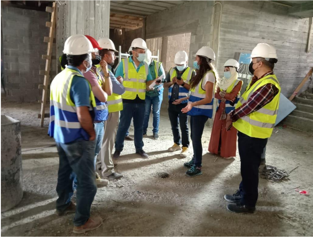
Aluminum work issue and Mechanical submittals were discussed with the Contractor
