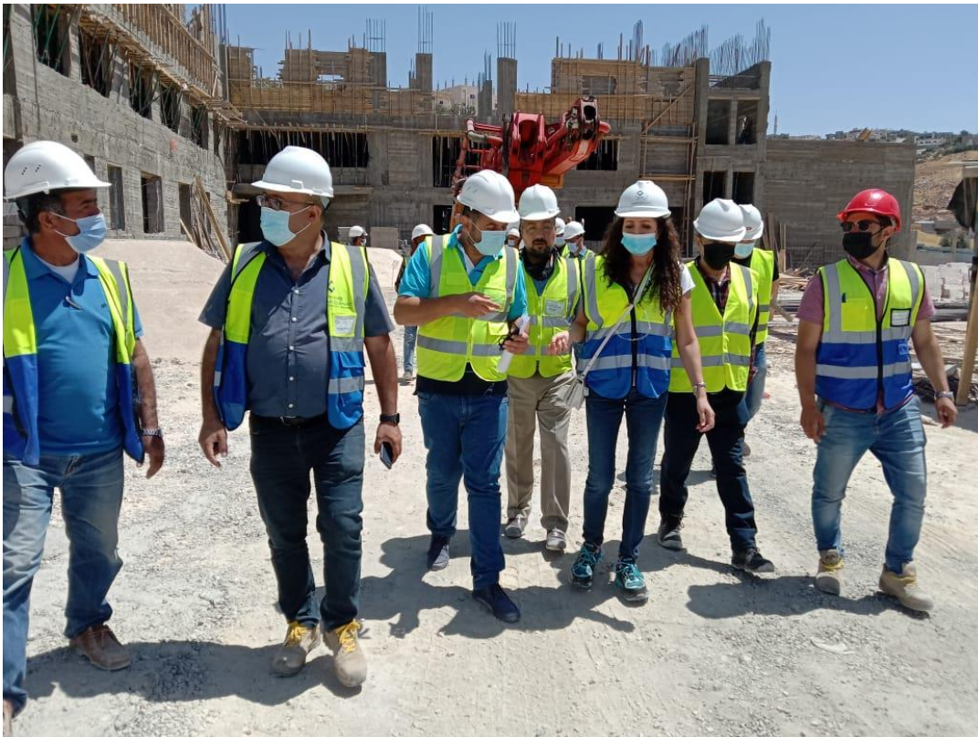
Tour inside the site was conducted
