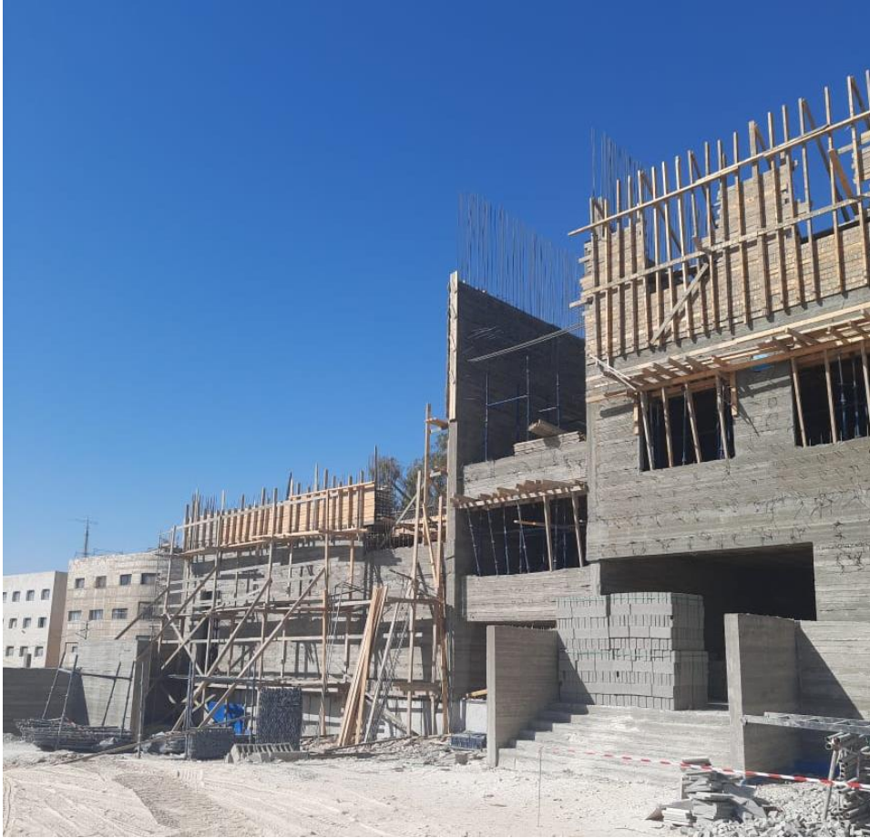
Formwork for external walls behind stone
