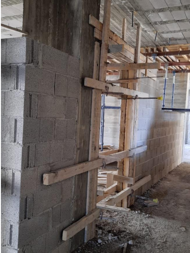
Formwork for door jambs and lintels
