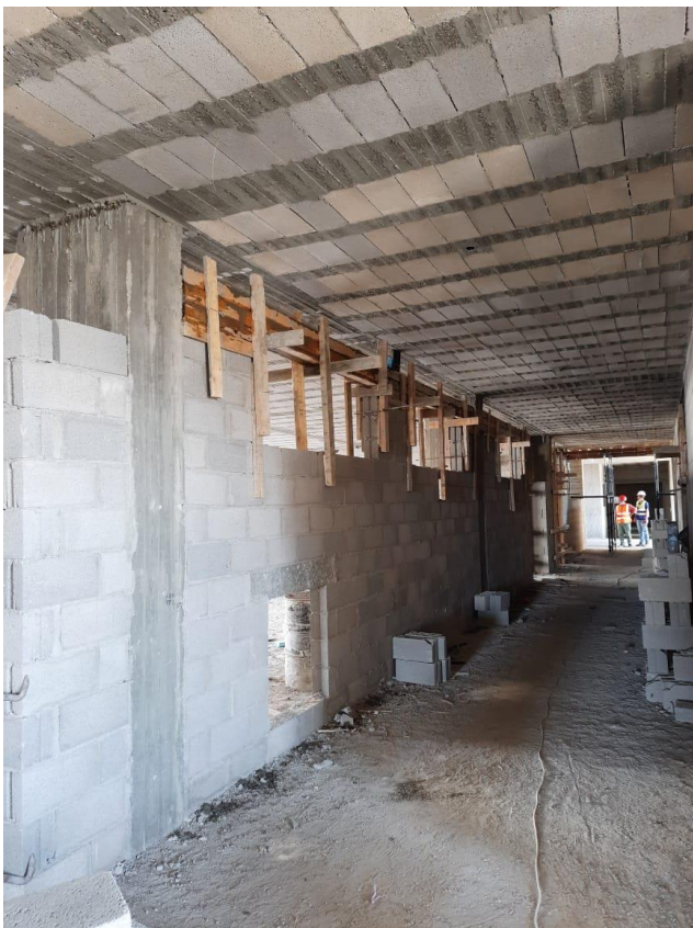
Formwork for lintels of internal windows
