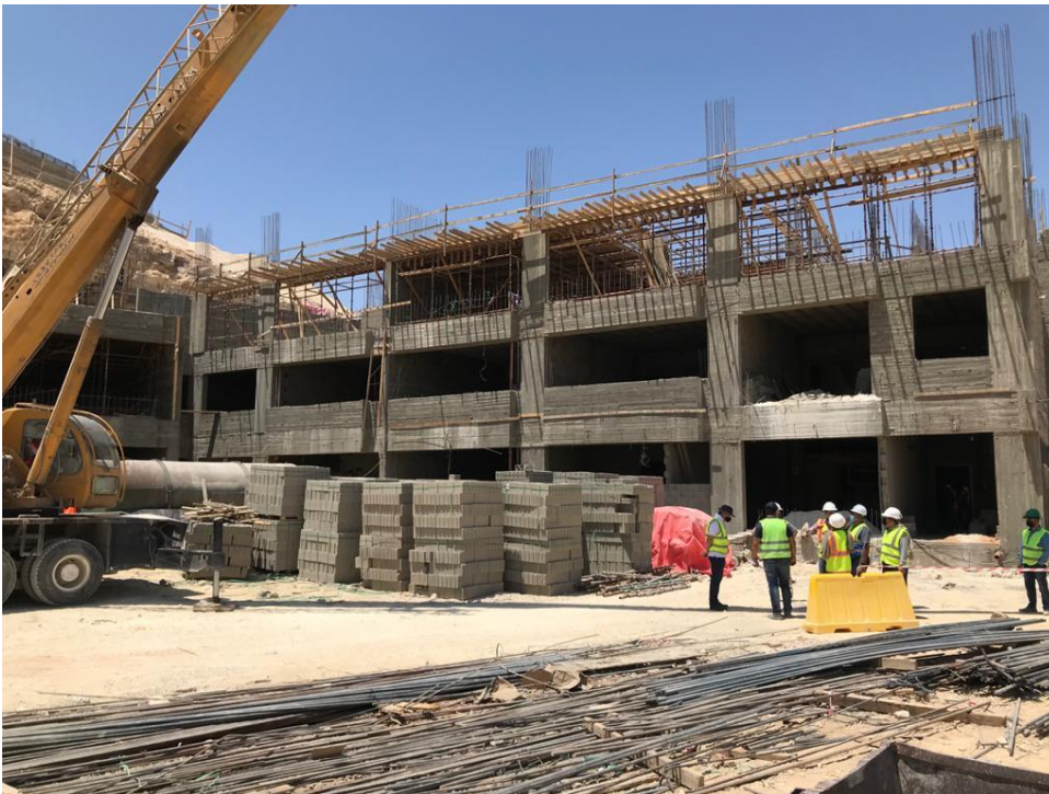
Starting of third floor slab formwork
