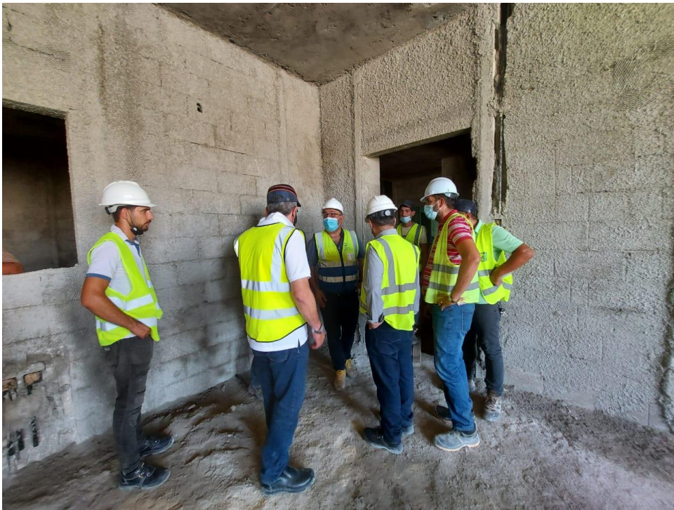
The quality of blockwork is acceptable
