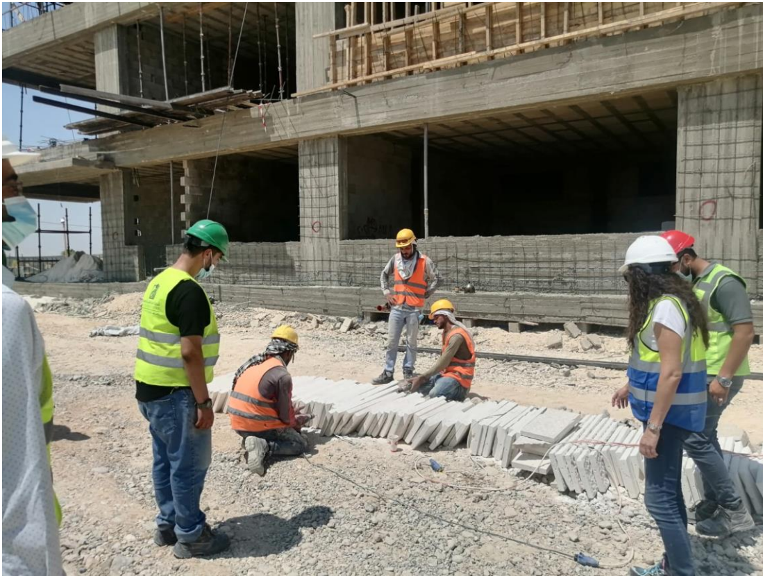
Preparing the stone for fixation at the facades
