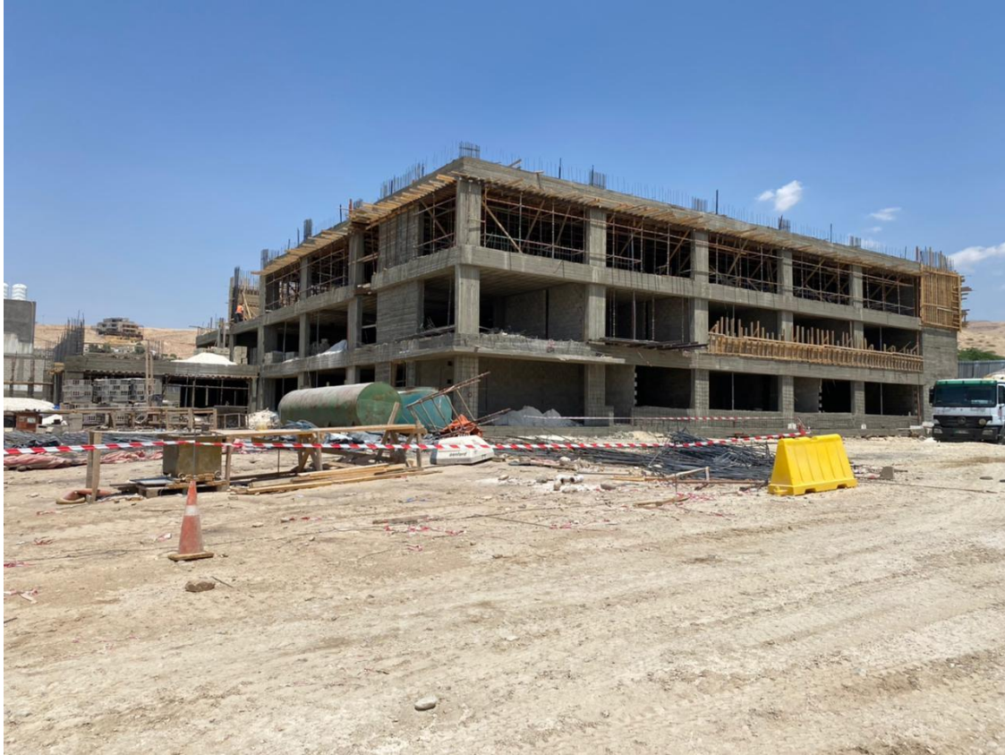
General view of the casted slab of the third floor
