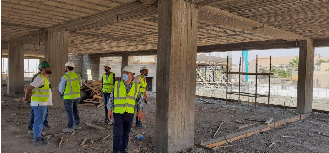
De-shuttering of the formwork of roof slab
