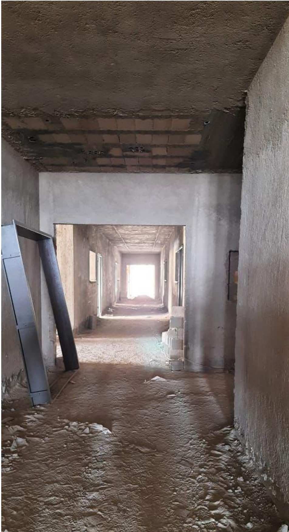
Plastering work at ground floor Zone "A"
