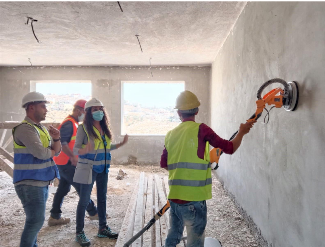
Final Coat plastering
