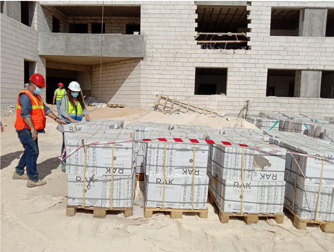
The Supervision team inspected the imported porcelain floor tiles
