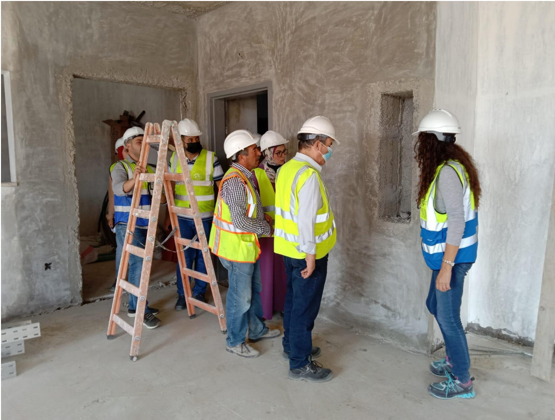
The supervision checked the location of the fire extinguishers in general
