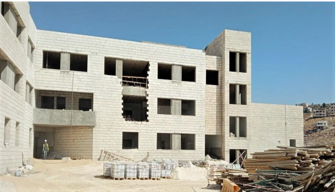
General check of the stone facades and window stone lintels
