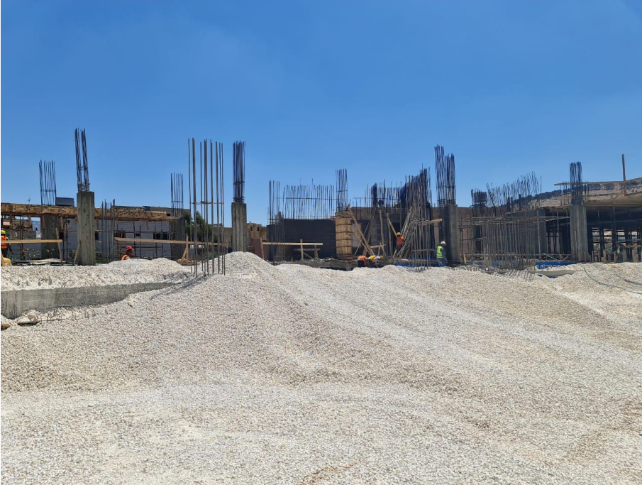
Checking the quality of Backfilling works at zone B
