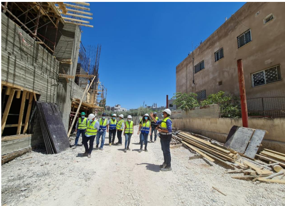
Checking concrete walls behind stone at zone A
