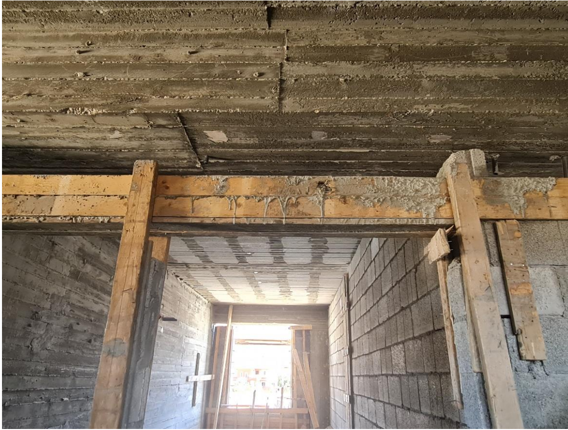
Doors' lintels casting
