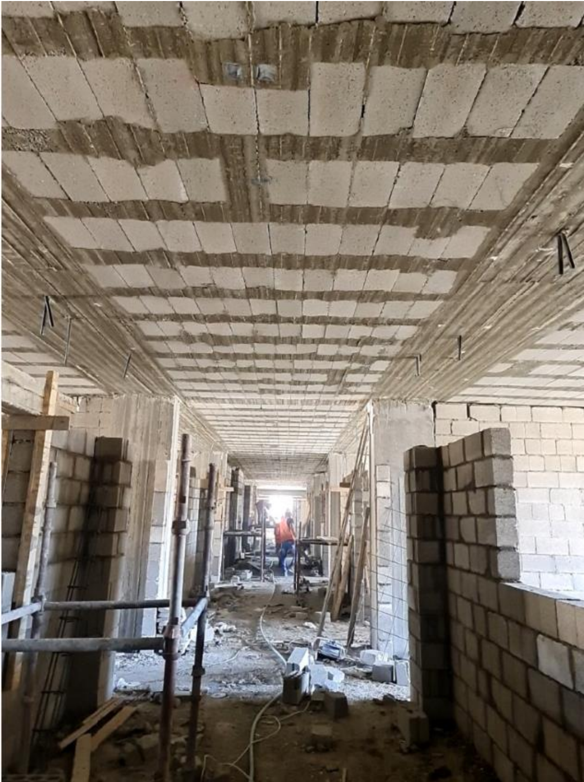
Blockwork have been checked at ground and first floors
