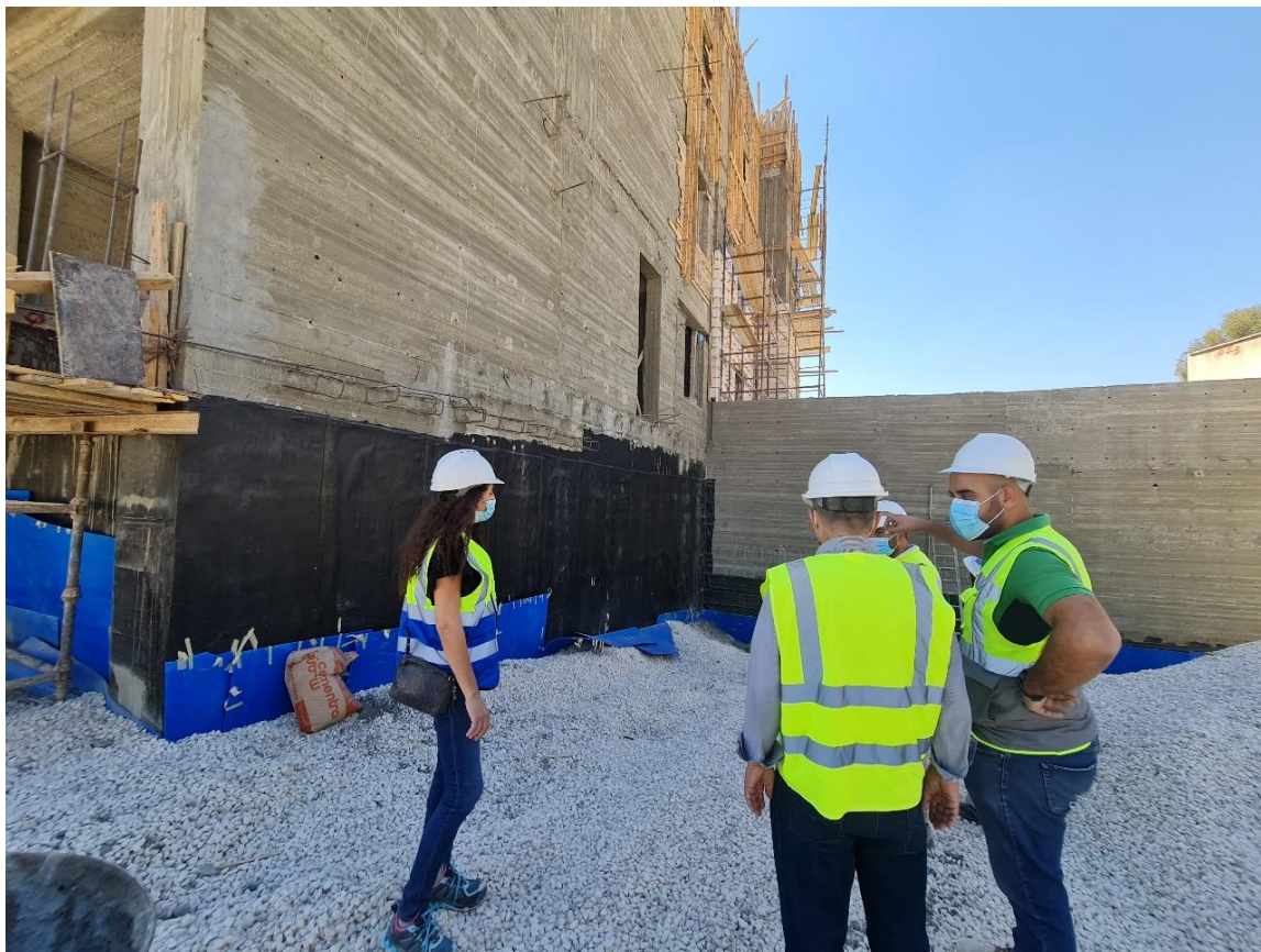
Remedy works were done by the Contractor
