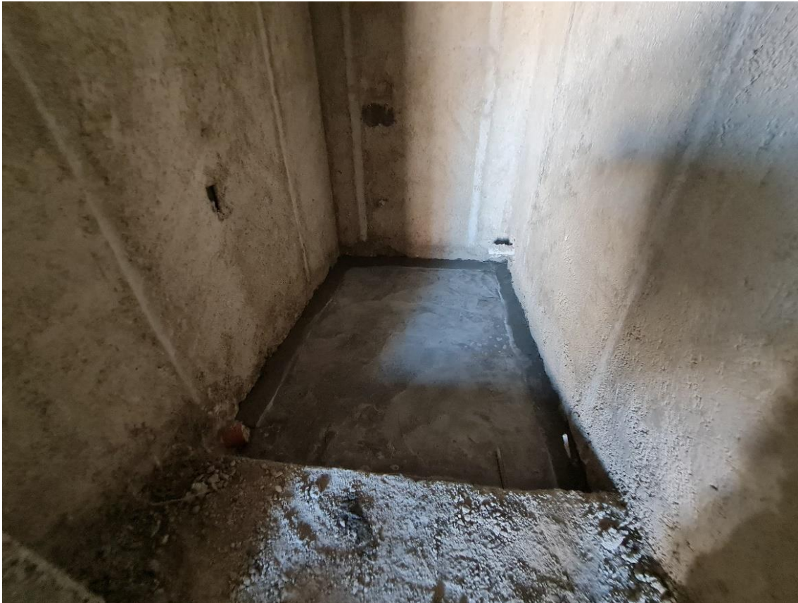
Executing first layer of insulation at the toilets' floor recess
