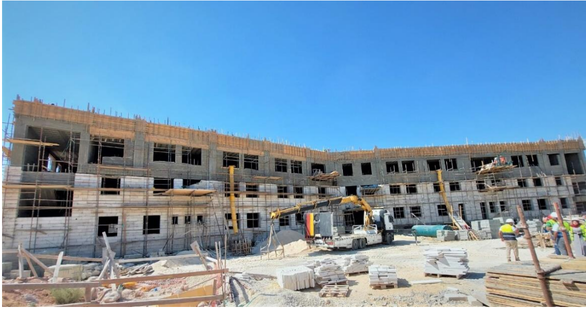
General view Preparing roof floor slab for casting (the last slab)
