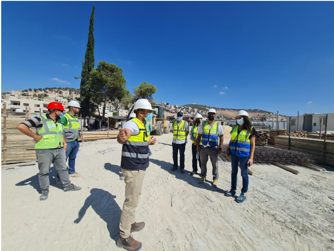
The Consultant's site engineer gave a brief about the ongoing activities
