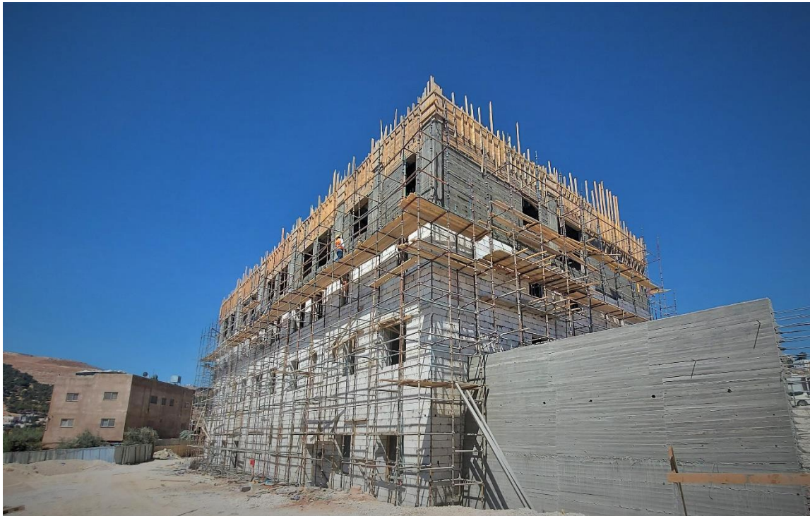
Checking the quality of executed stone works at school elevation
