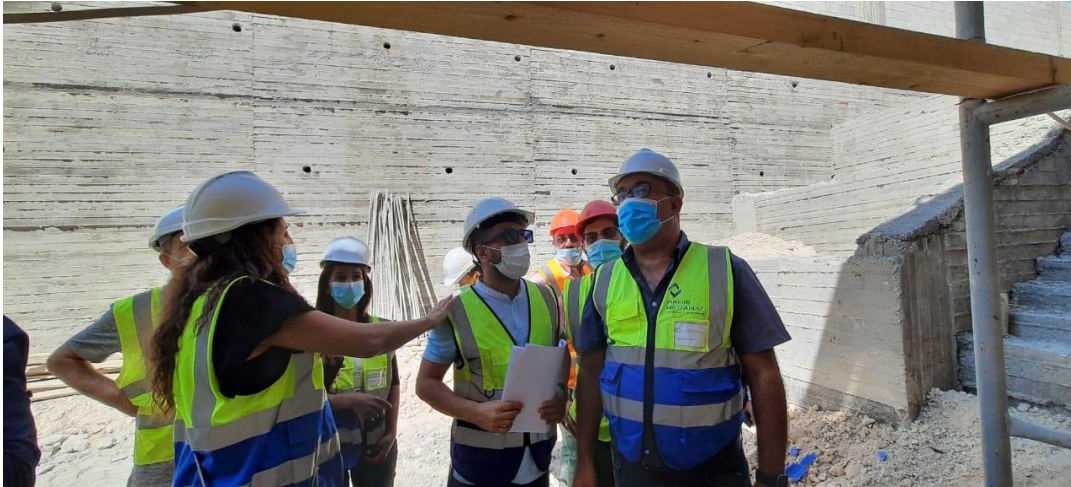
Yousef Omar/ supervision site engineer gave a brief on work progress, the current stages and the function of each part
