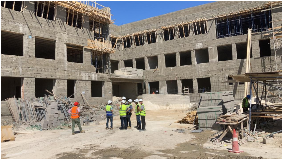
The quality of concrete work is acceptable in general
