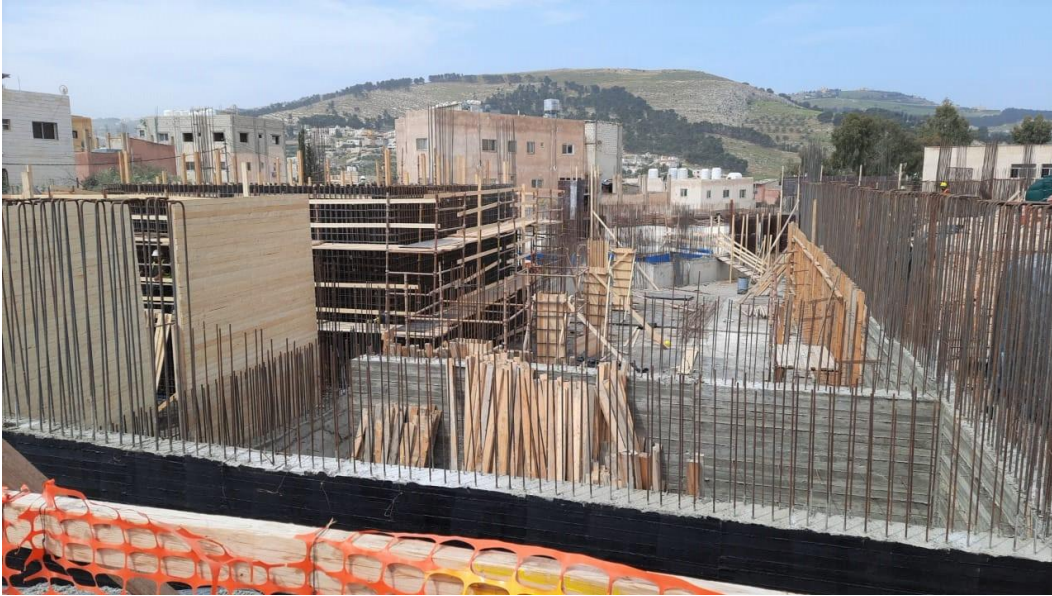
General view of the site.
