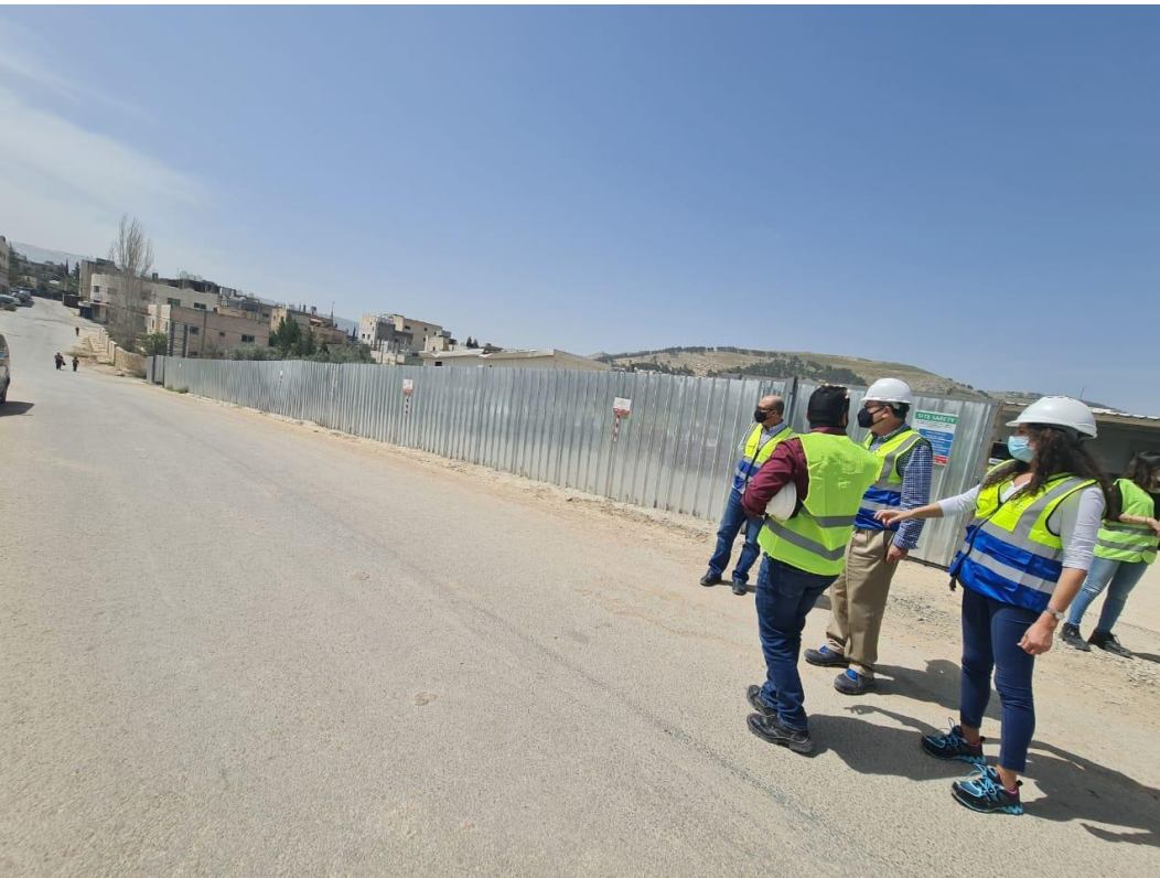
There is an encroaching of neighbor wall towards the school boundary plot.
